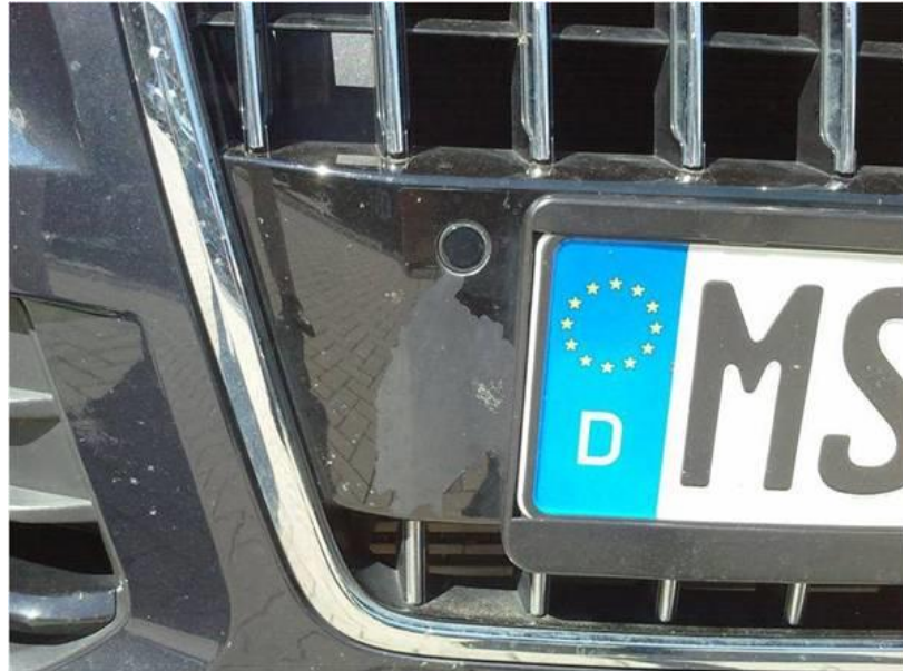
Figure 1. Example of flaked-off paint.
