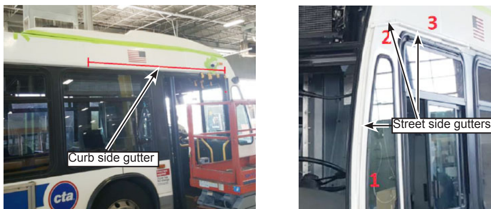
Figure 43 - Install the Gutters
