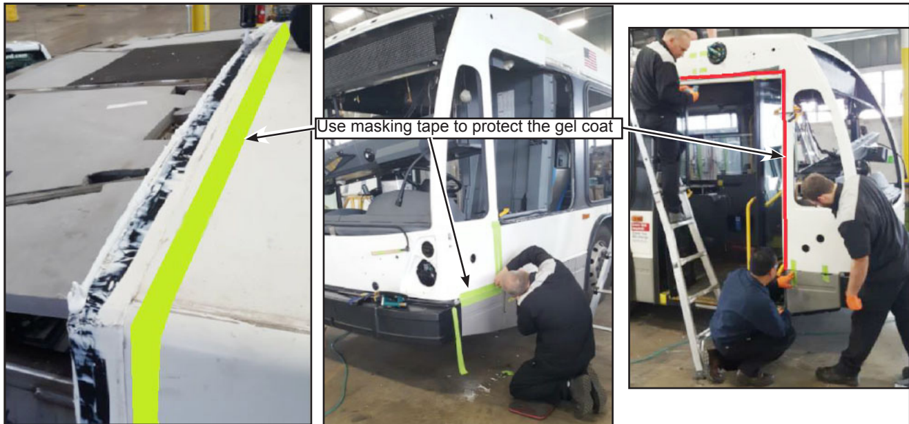
Figure 27 - Protect GelCoat with Masking Tape
