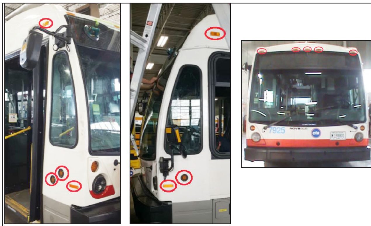
Figure 47 - Install Reflectors, Marker Lights and Signal Lights
