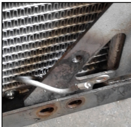
Figure 4 - Typical View of Ground Cable Connection
