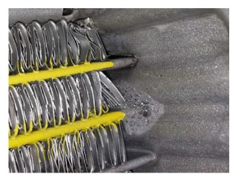
This condition may be the result of excessive thermocycles within the cooling system caused by excessive cycling of the thermostat. These excessive thermocycles within the coolant system may cause the tubes to fatigue, crack and leak at the radiator headers. To correct this condition, a new thermostat has been designed that eliminates the thermostats excessive cycling.
