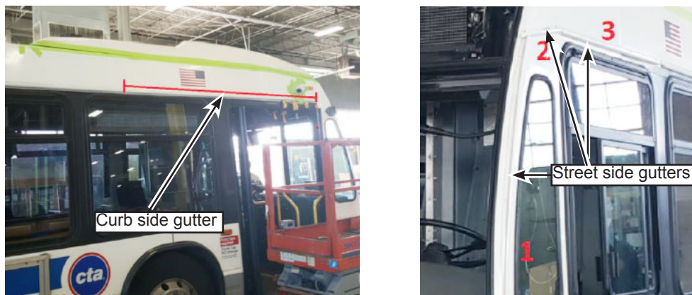
Figure 43 - Install the Gutters
