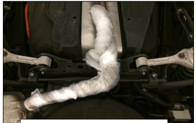
Exhaust near rear cross member
