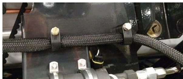
Figure 6: Stauff clamps main fuel line routing
