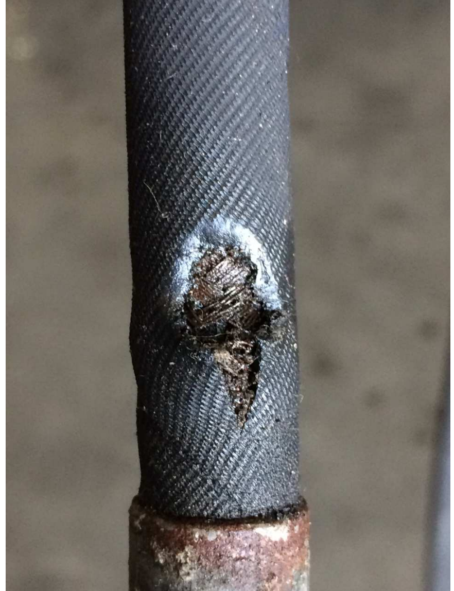
Damage being caused
