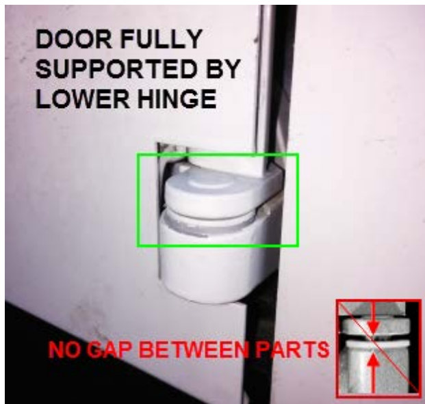
FIG.6 LOWER HINGE SUPPORT
