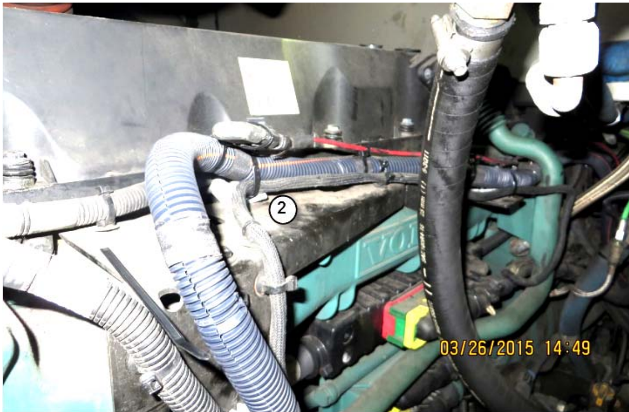
FIGURE 15: POWER CABLE ATTACHED TO #2 DOUBLE-TIE MOUNT AND PROPER NYLON TIES INSTALLATION
