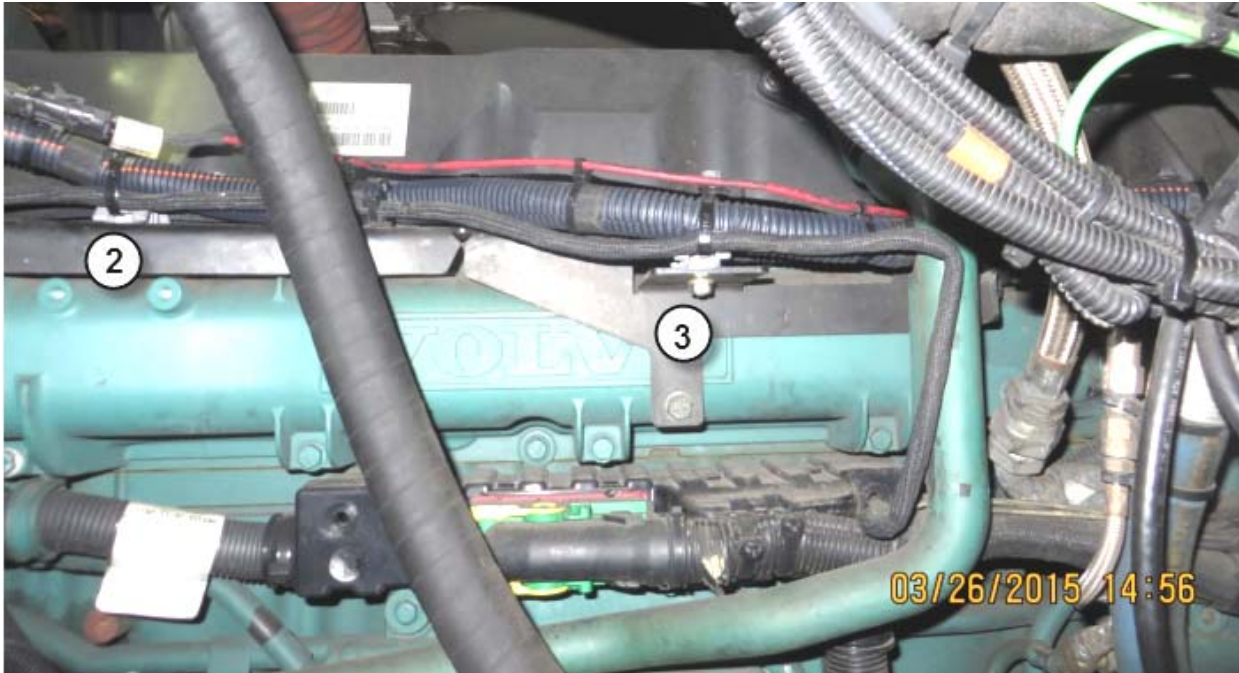
FIGURE 16: POWER CABLE ATTACHED TO #2, #3 DOUBLE-TIE MOUNT AND PROPER NYLON TIES INSTALLATION
