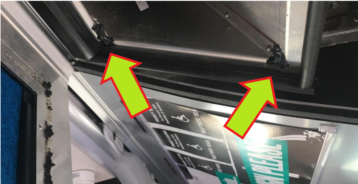
Figure 5: Seal duct corners with sealant
