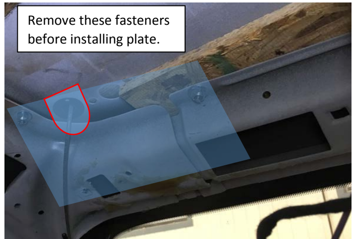
Figure 3 Roof reinforcement area with nuts that need removed.
