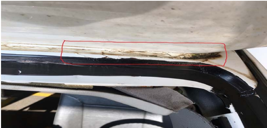
Figure 1 The area inside the red box will need sealant removed.
