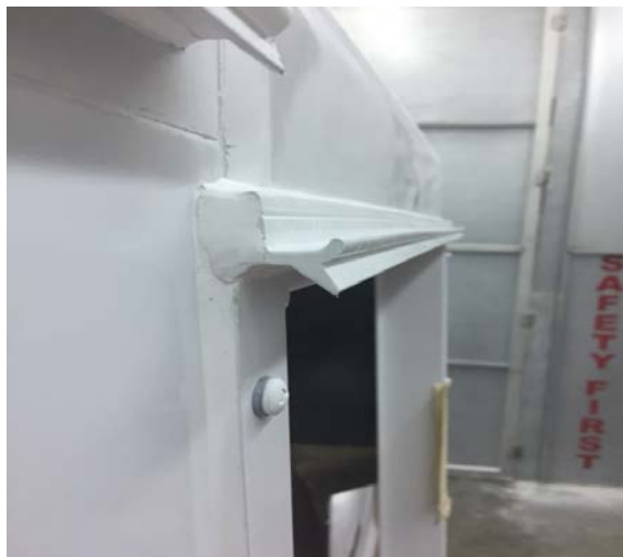
Figure 6 Drip rail placement and appearance for reference.
