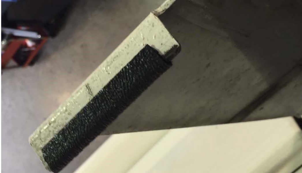
Figure 5 Example of installed edging. This is the short piece at the corner of a door.
