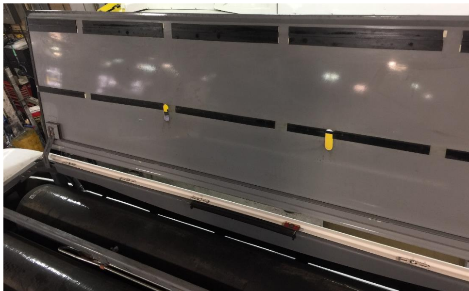
Figure 8 The rubber strips are cut into sections to simplify installation and replacement as the rubber wears. Actual length is not critical, but a suggested gap is 2-inches between strips as shown.
