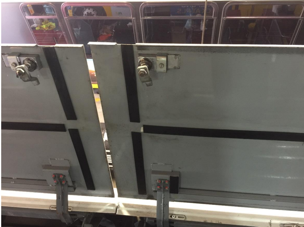
Figure 7 The door surfaces are cleaned and prepared for the adhesive, and the new rubber strips are installed in the locations touching the system frame.
