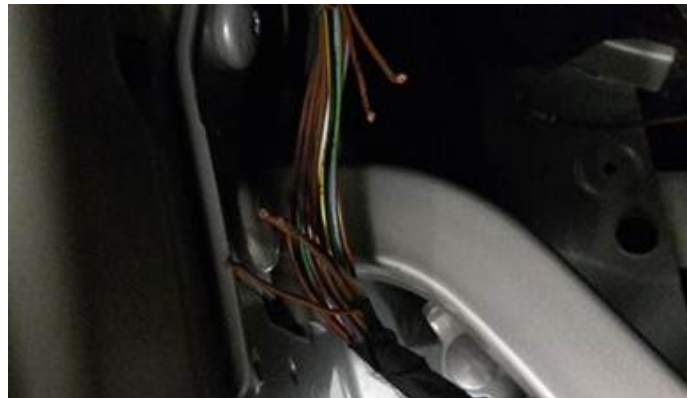
Figure 1. Wire damage at trunk hinge.
