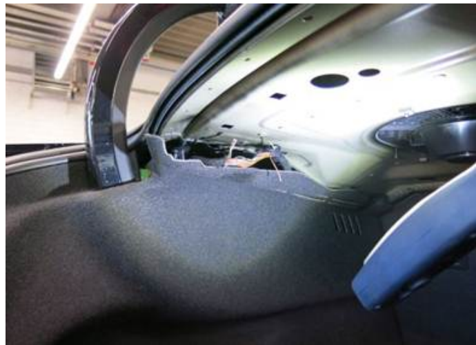
Figure 2. Wire damage at trunk hinge.
