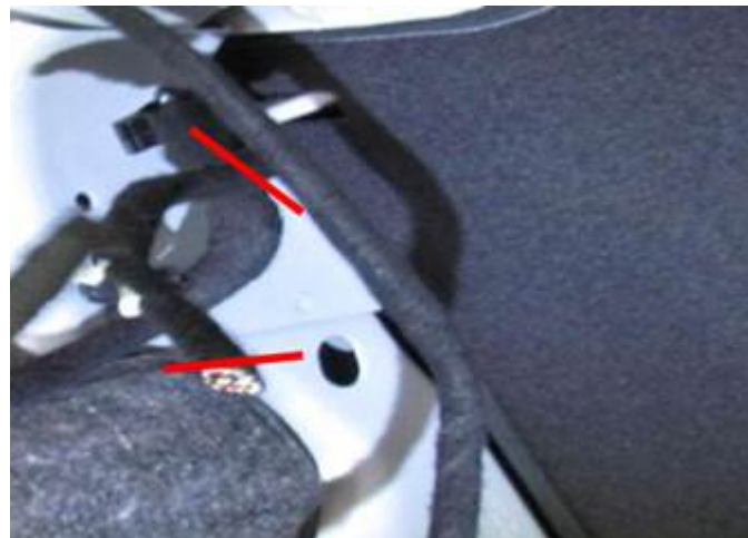
Figure 10. Open the winding of the cut-off vehicle wiring harness to the junction of the main harness on separable area (red marks).
