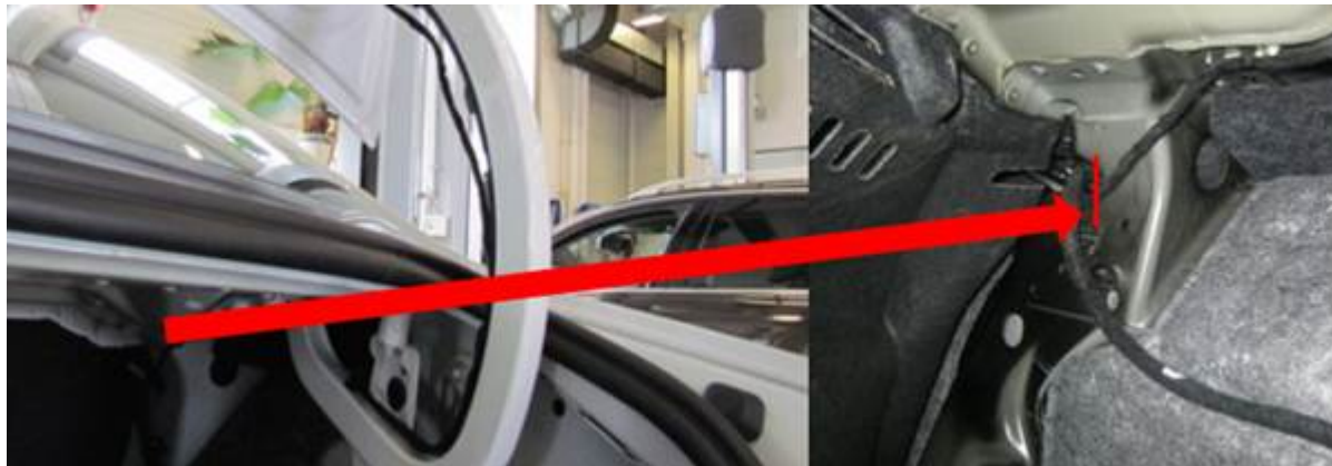
Figure 2. Cut cable off on the junction of the main wiring harness (red separation line).
