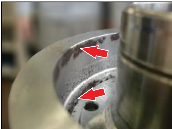
Figure 8. Rust/Corrosion on Inside of Coupling Body
