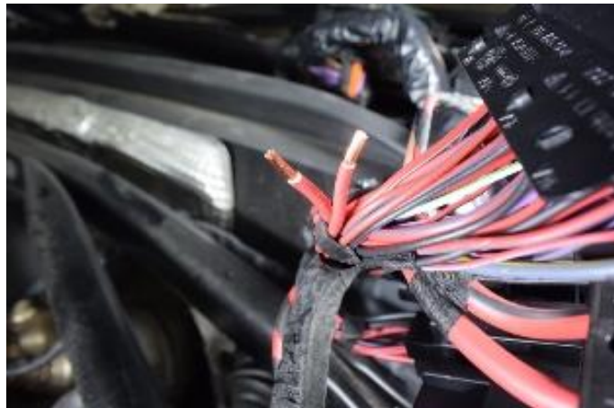
Figure 19. Stripped wire ends.
