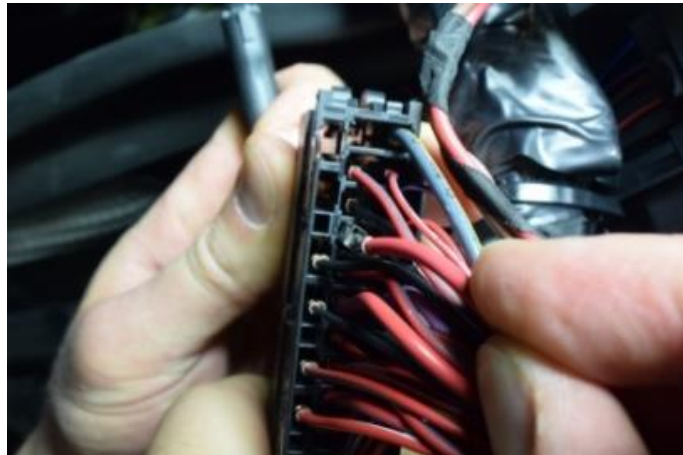
Figure 16. SB4 battery power feed wire.
