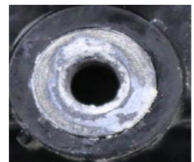
After wire brushing
