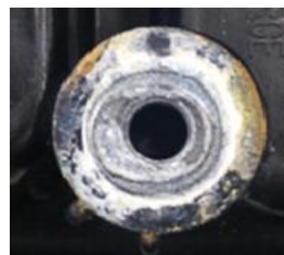
Before wire brushing
