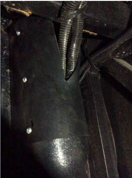
Reinstalled Hydraulic Lift Cover
