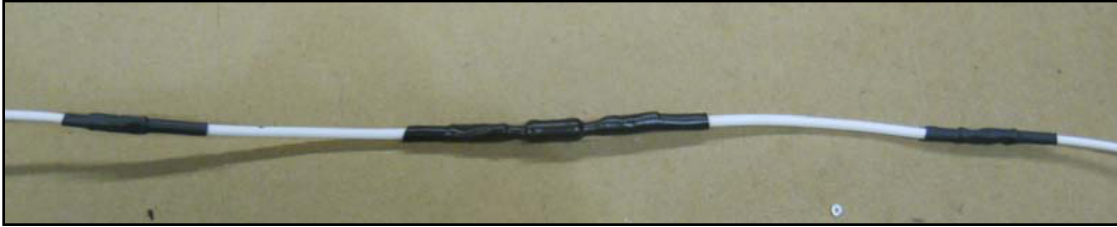
Figure 8 - Typical View of Jumper Harness (N8902748) with Splice Covered
