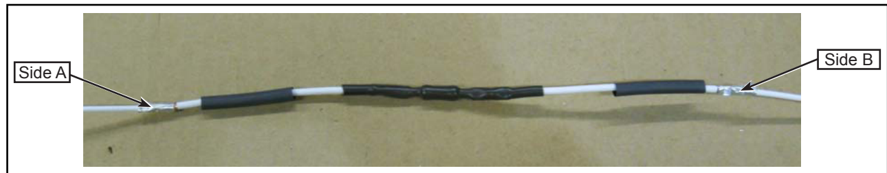
Figure 7 - Typical View of Jumper Harness (N8902748) Connected on Each Side
