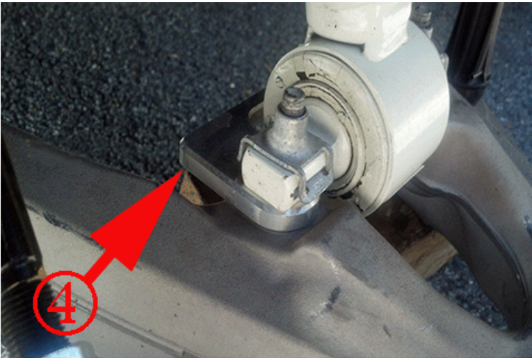
4. Aftermarket lift kit blocks installed
