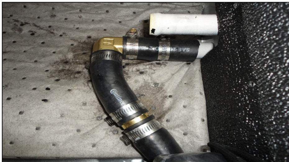
Figure 10, Installation of 4 inch lines onto elbow
