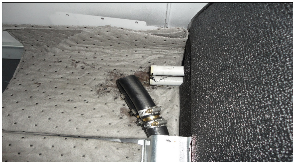
Figure 7, Installation of 4 inch hose and brass fittings
