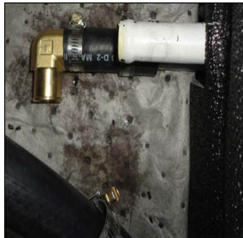
Figure 9, Installation of elbow on Davenport tubes
