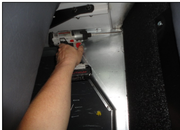
Figure 3, Removal of interior heater hose cover
