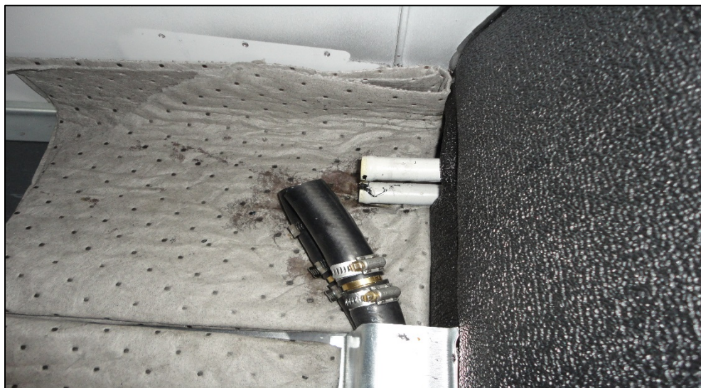
Figure 7, Installation of 4 inch hose and brass fittings
