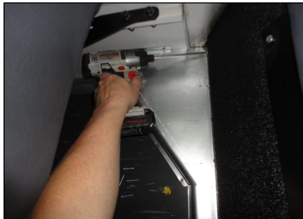
Figure 3, Removal of interior heater hose cover
