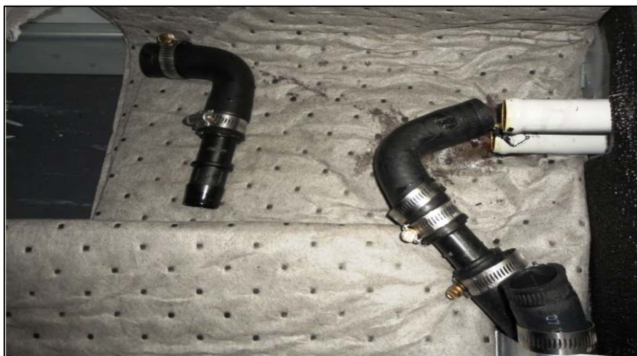
Figure 6, Removal of rubber elbow
