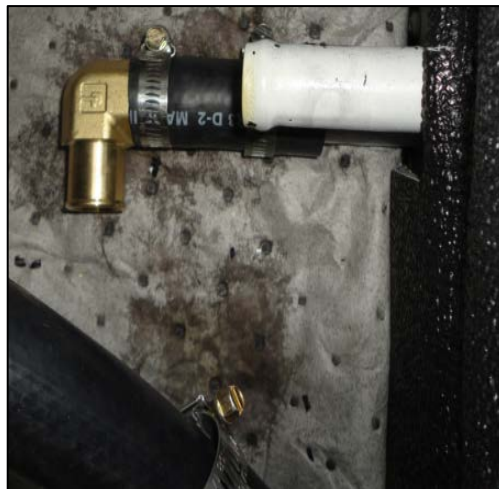
Figure 9, Installation of elbow on Davenport tubes
