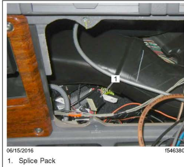
Fig. 14, Splice Pack Located Behind the Auxiliary Instrument Panel
