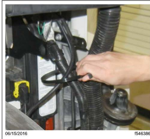
Fig. 6, Securing Wire 433 with a Cable Tie
