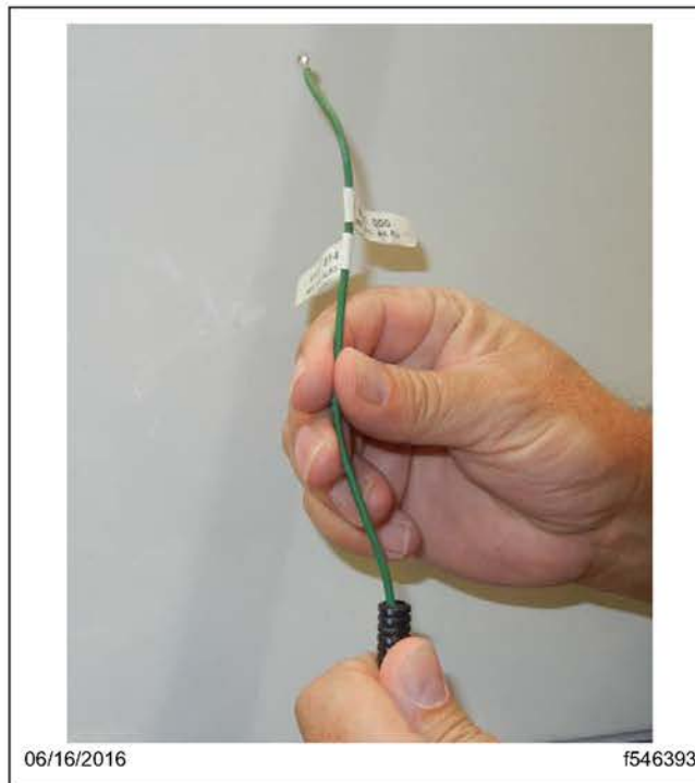
Fig. 3, Feeding Wire A06-91061-000 into the Conduit
