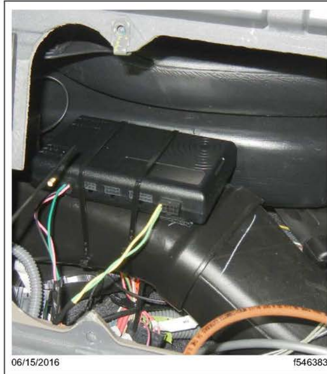
Fig. 15, Virtual Technician Secured with Tie Straps
