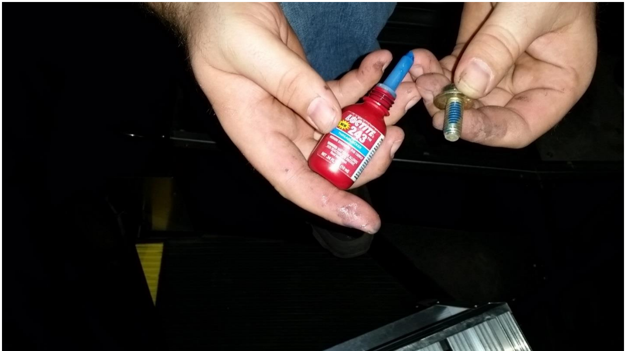
Figure 18: Apply Loctite to the bracket bolts
