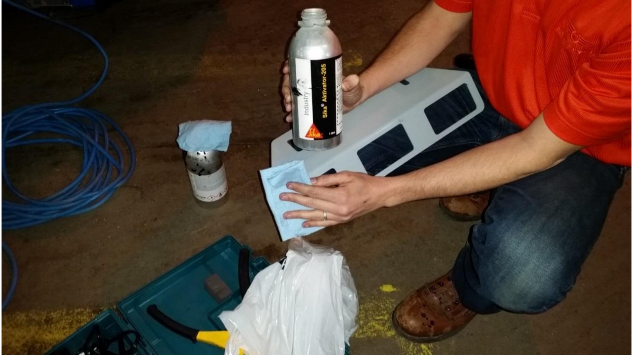
Figure 7: Apply Sika Aktivator/Cleaner on the bonding surface of the bracket
