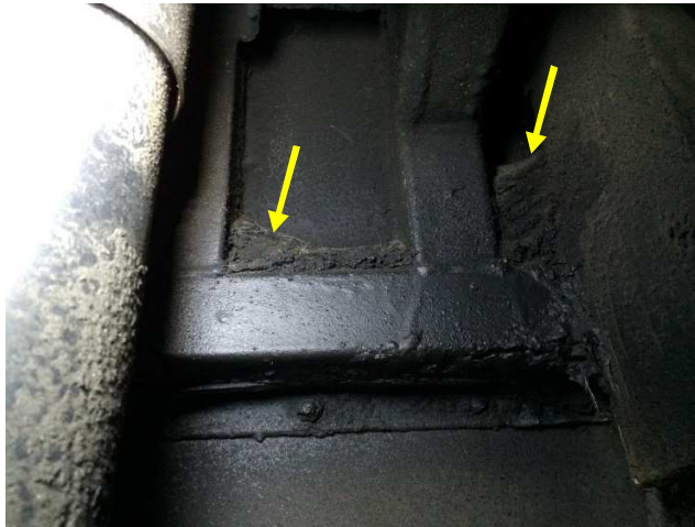
Figure 1: Road debris and salt built up on underbody structure
