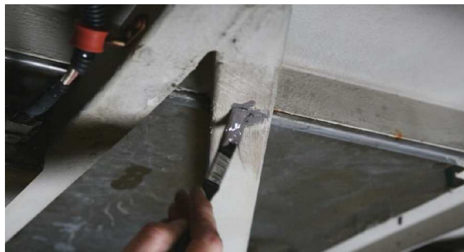
Figure 12: Apply zinc primer to the underbody structure with a brush
