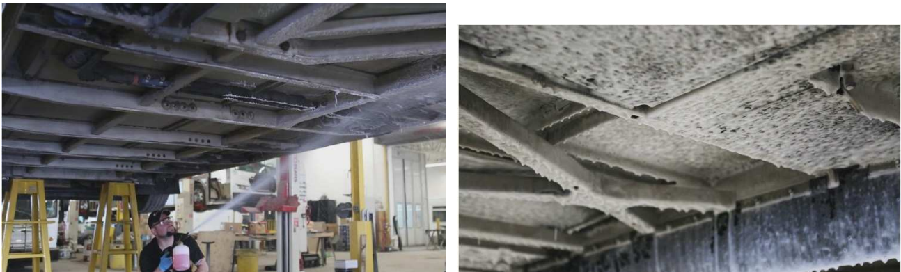
Figure 8 and 9: Spraying Salt Eliminator and foam built up on underbody structure
