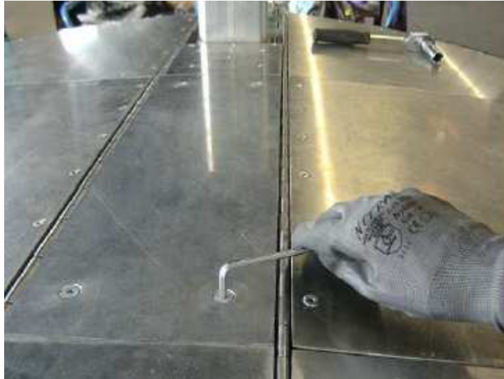
Figure 1: Top plate on the top of center cross beam
