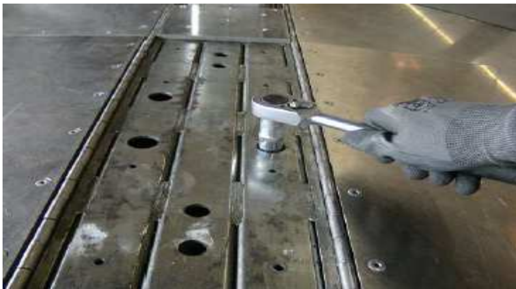
Figure 4: Top center cross beam nuts/bolts
