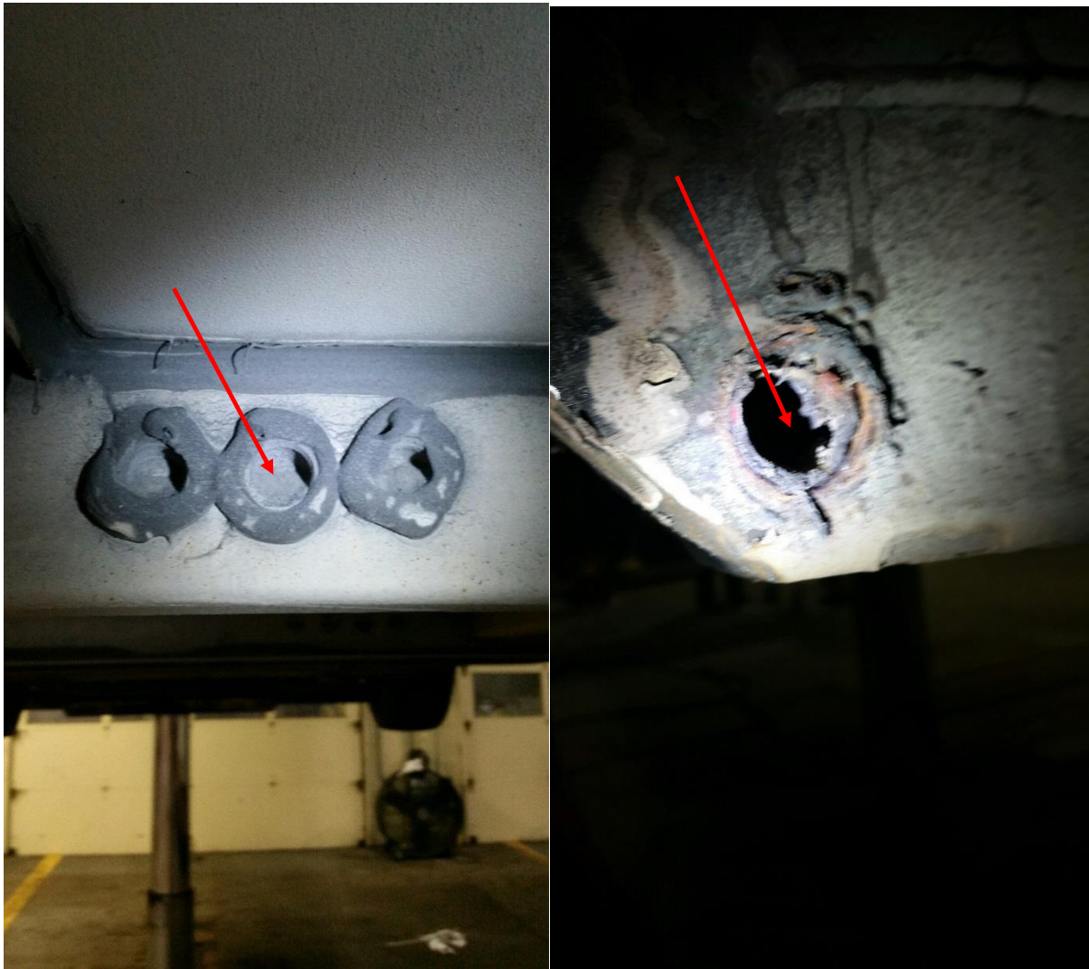
Plug to be cleaned out & inspected for cracks
