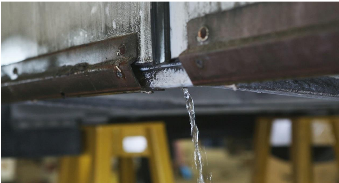
FIGURE 13: WHEN WATER COMES OUT CLEAR, THIS IS A GOOD INDICATION THAT DEBRIS AND CALCIUM HAS BEEN REMOVED FROM THE INSIDE OF THE TUBES.
