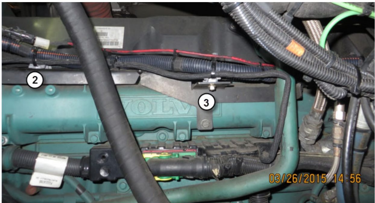
FIGURE 13: POWER CABLE ATTACHED TO #2, #3 DOUBLE-TIE MOUNT AND PROPER NYLON TIES INSTALLATION
