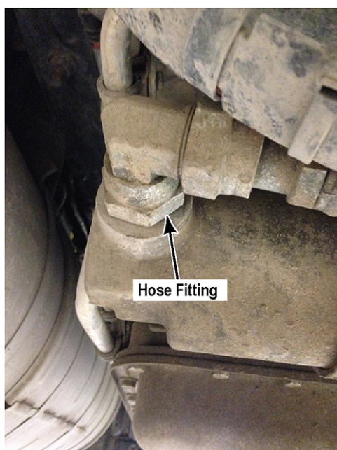
Cooler return line
