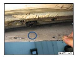
7. Properly deburr both sides of the drilled hole.
