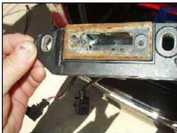
Figure 2 – Corrosion around License Plate Light
