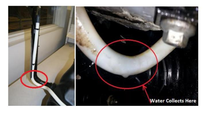
If the vent path is blocked or restricted, install a Shepard's crook (U-shaped) vent to stop moisture from entering the vent line.
