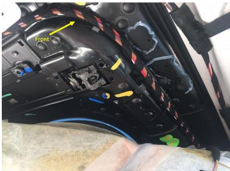
Figure 1 (Water leaking through corner of water channel)
