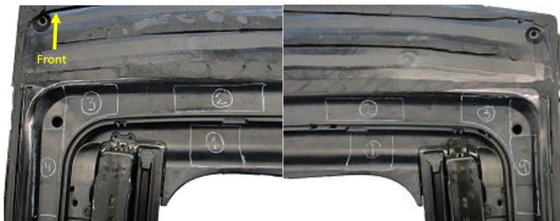
Figure 3 (Inspections zones for stress cracks / application zones and sequence for foil application)
