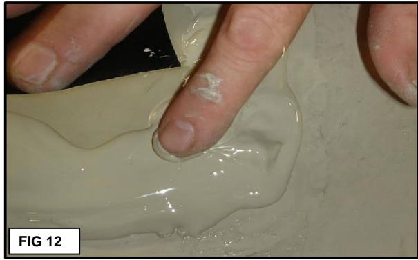
Fig 12: Close voids or pinholes by gently swirling your finger in a small circular pattern, gradually lifting your finger
