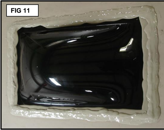
4 Fig 11: Finished skylight with new sealant applied.
