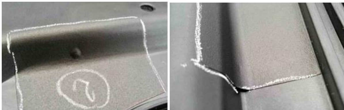
Figures 23 and 24 Air bubble under foil, air gap underneath foil.
