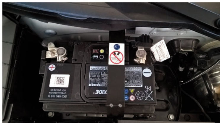
Option I194 60Ah battery installed in vehicle.
