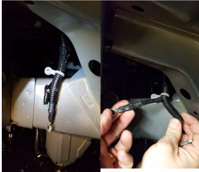
Fig. 7 Removing Tape From Conduit
