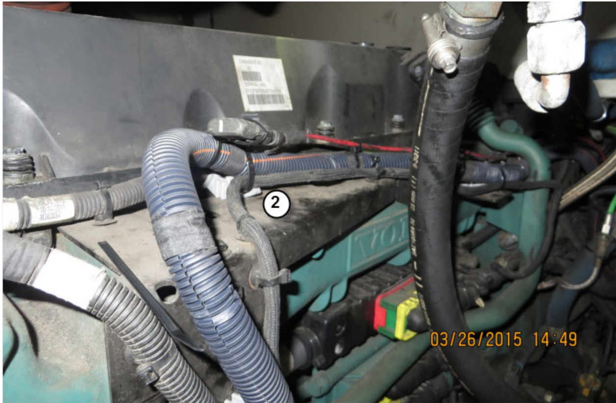
FIGURE 12: POWER CABLE ATTACHED TO #2 DOUBLE-TIE MOUNT AND PROPER NYLON TIES INSTALLATION
