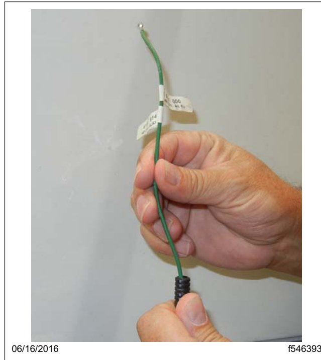
Fig. 2, Feeding Wire A06-91061-000 into the Conduit
