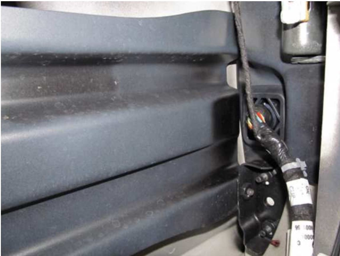
This can also occur in the front and/or rear area of the door beam; with the condition sometimes more evident in the front area (shown above) where the radio speaker is mounted.
