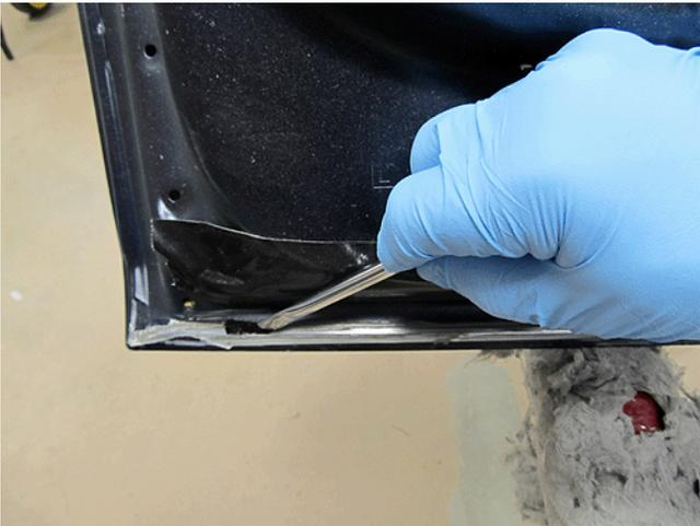
7. Using \*Lloyd's Pure Prep™ Metal Surface Preparation P/N 25418 (10 fluid ounce bottle) in a spray bottle, saturate the complete flange area with the pre diluted solution and scrub the area well, rendering a foaming of the Pure Prep.™ This will greatly improve adhesion and corrosion resistance in the repair areas.
