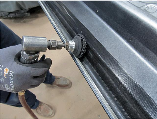
If sand blasting is not available, remove the rust using a 3-M Scotch-Brite™ Clean and Strip Disc, Part # 07466, abrasive wheel.
