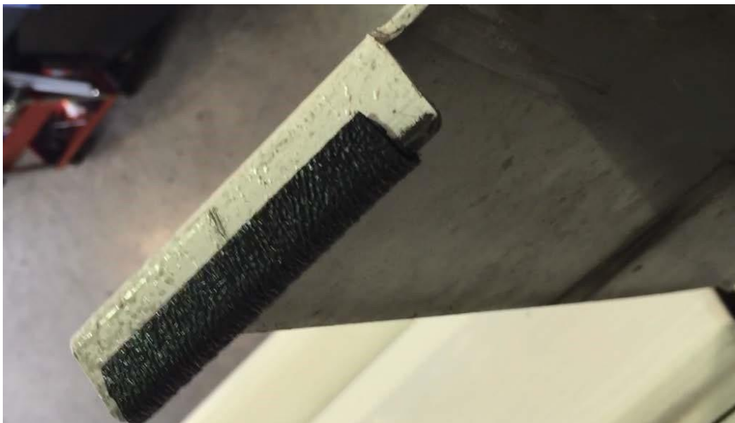
Figure 9 Example of installed edging. This is the short piece at the corner of a door.
