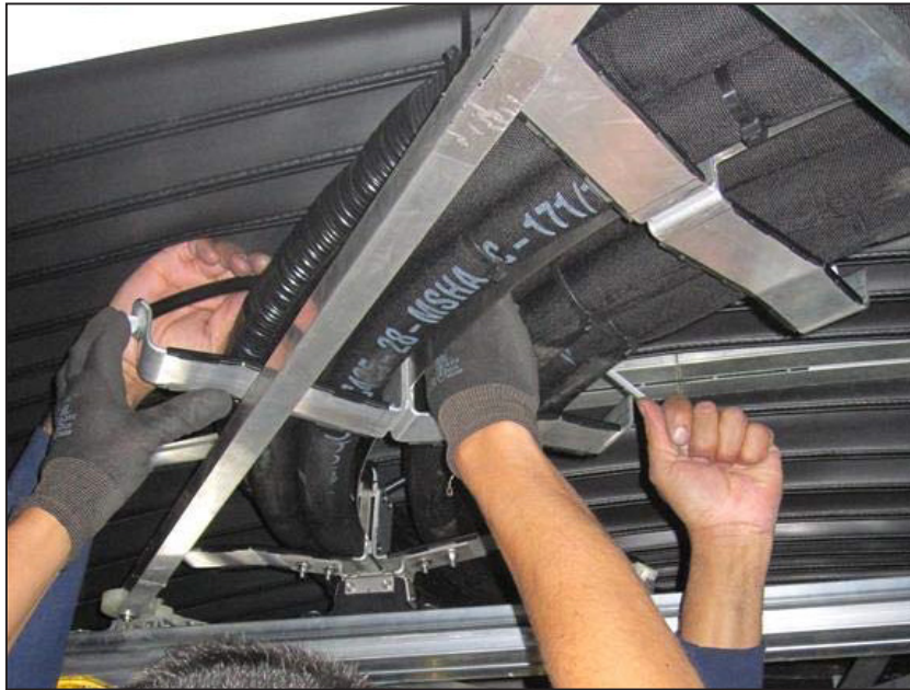
Figure 8 - Spacing Tubes Installation
