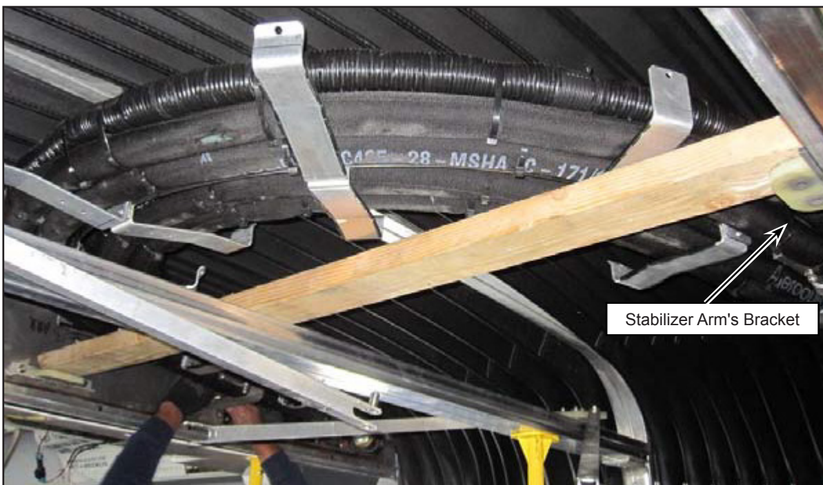
Figure 6 - Wood Piece Installation
