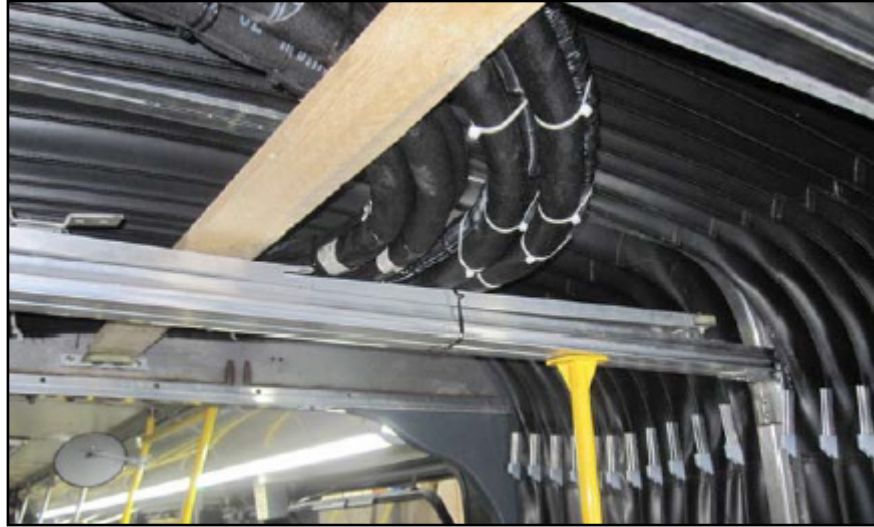
Figure 14 - Install the New Guiding Profile
