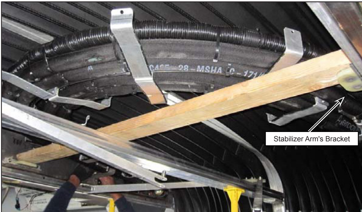
Figure 6 - Wood Piece Installation
