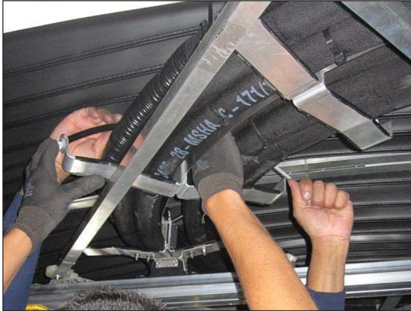
Figure 8 - Spacing Tubes Installation
