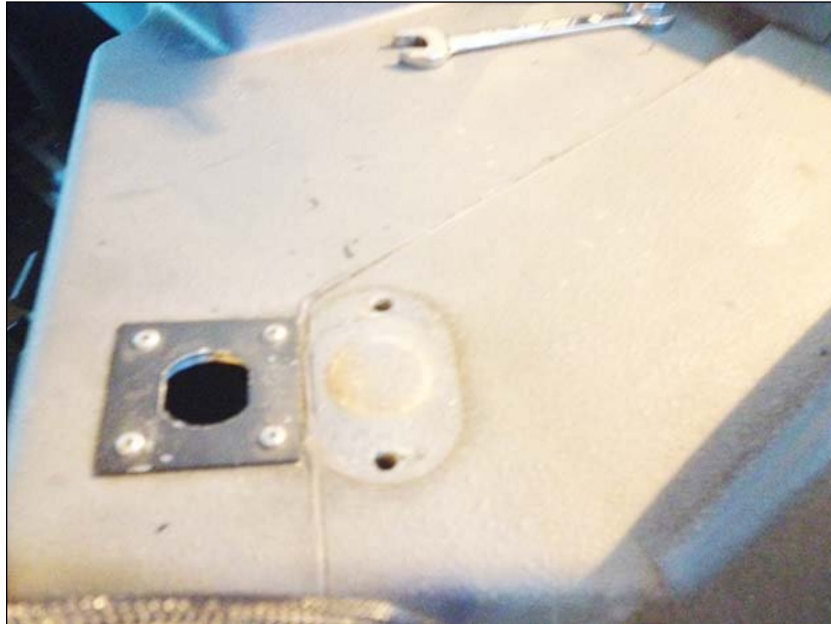
Figure 29 - Install Transfer Ticket Holder, NTP Wiring and Sealant
