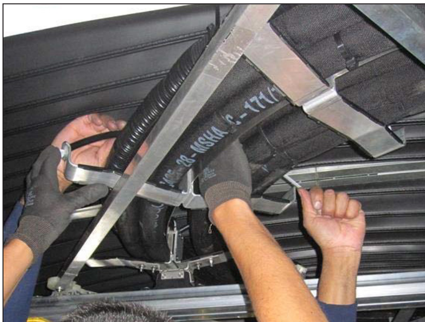
Figure 8 - Spacing Tubes Installation
