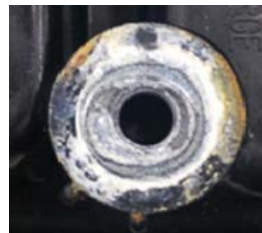
Before wire brushing
