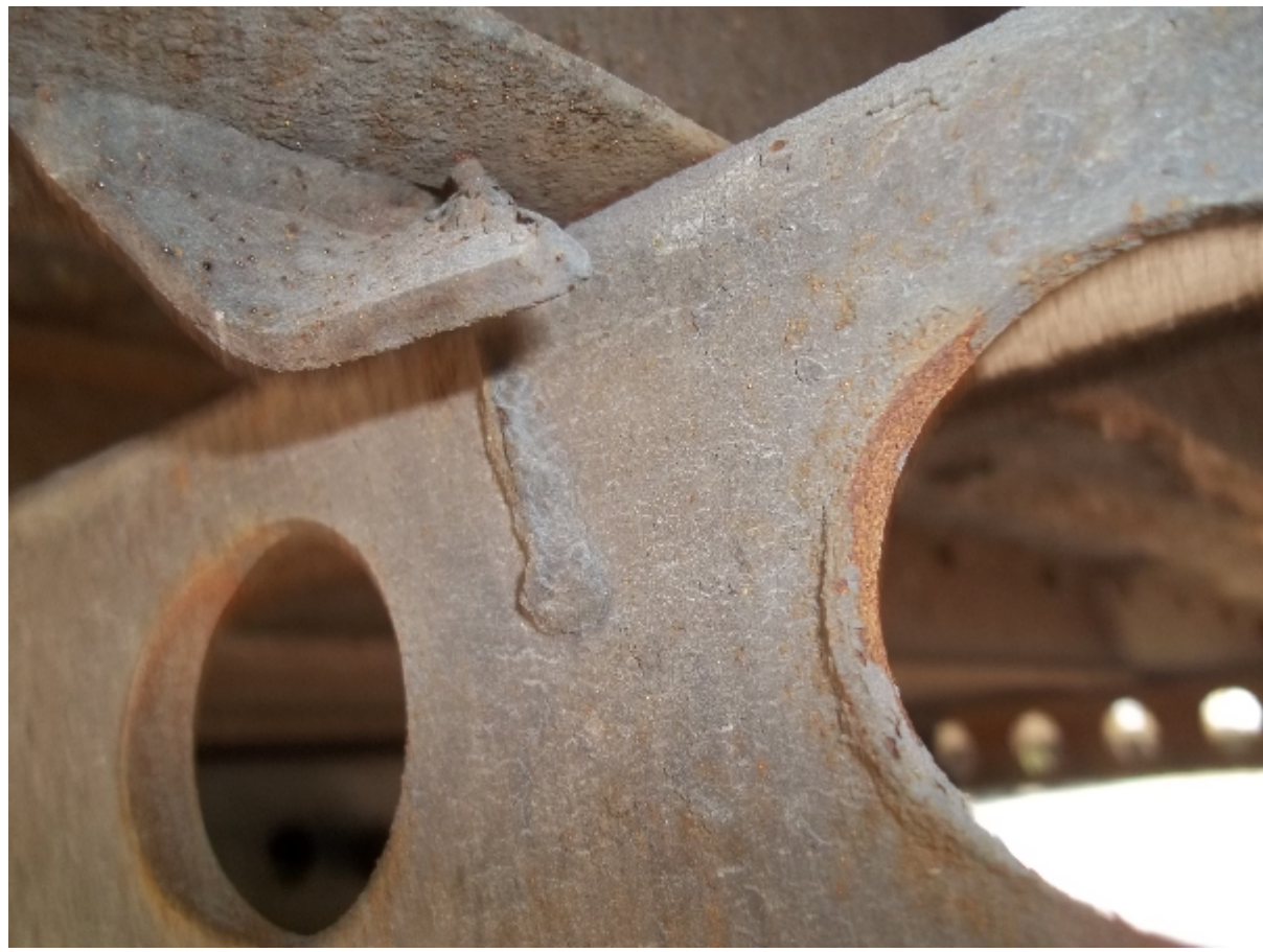
BENT/CRACKED GUSSETS
