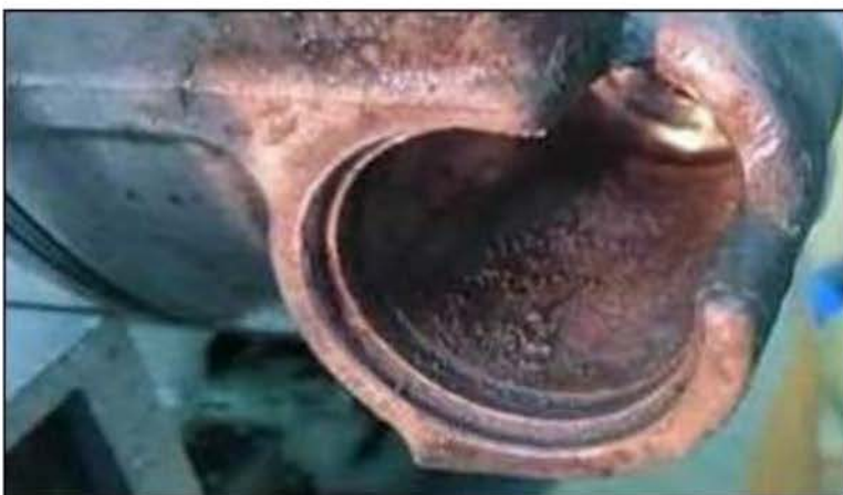
Figure 14. Corrosion in the N280 valve bore.
